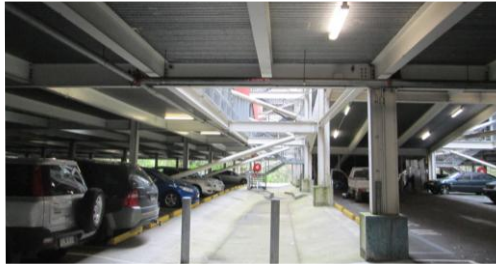
Deakin Carpark 6, Burwood
