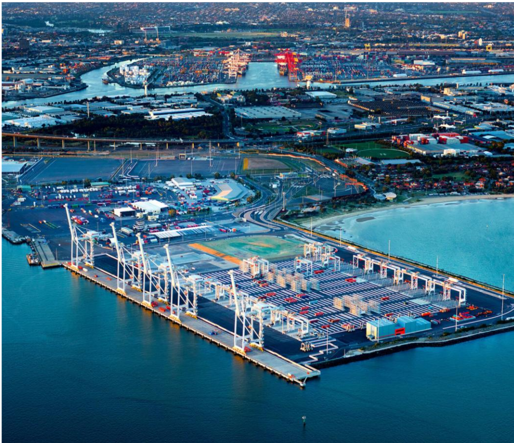
Webb Dock, Autocare Facility, Melbourne
