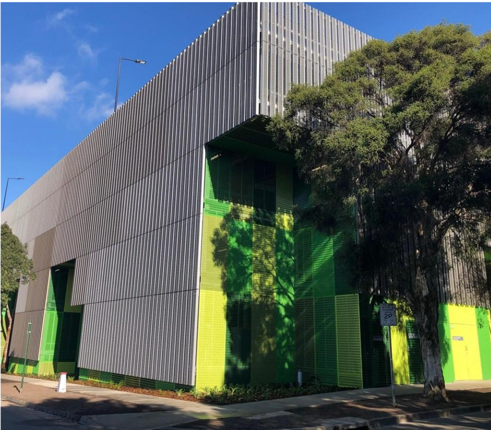
Harrow St, Carpark Box Hill
