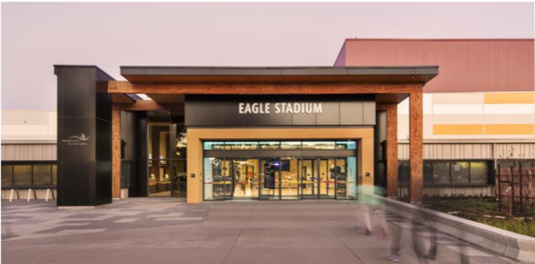
Eagle Stadium, Wyndhamvale
