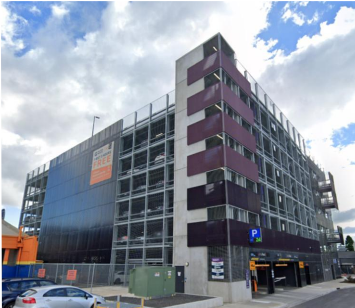
Brimbank Multi-Deck Car Park
