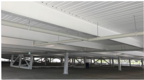
Deakin Carpark 12, Burwood
