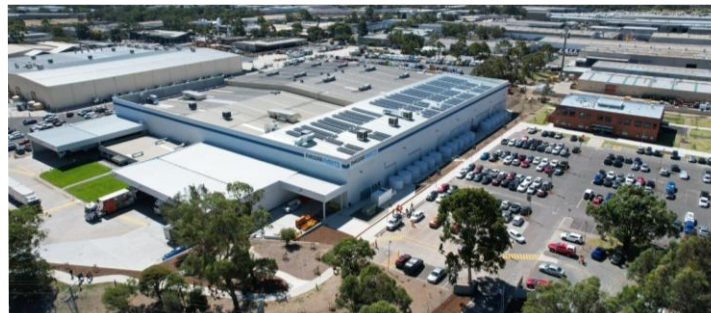
Paccar Parts Warehouse, Bayswater
