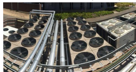
HVAC Asset Replacement, Deakin University
